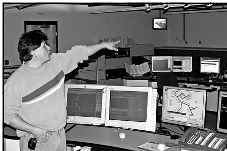
The state-of-the-art Mariposa Control Center, where a new system monitors and controls train movements and electrical power.
