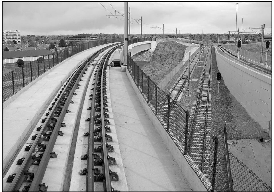
Two of the three levels of track on the grade-separated I-25 / I-225 interchange. – Photo © 2006 Bob Wilson.
