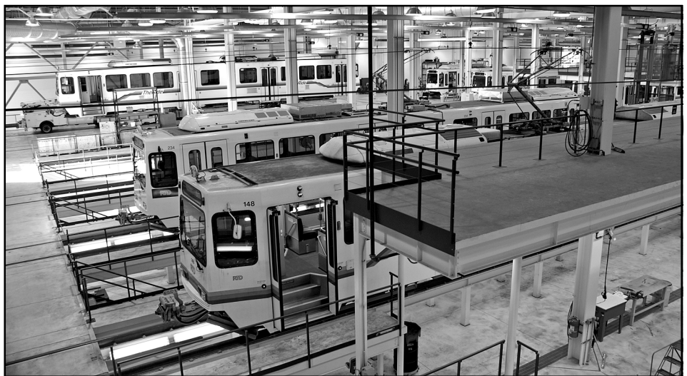
View of the modern Elati LRT maintenance bays. Note all the well-lit pits under the cars. Elati Maintenance Facility.
